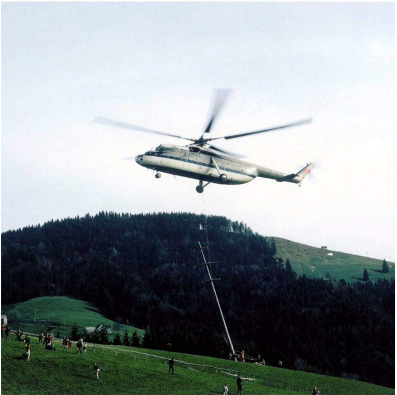
Herisau/AE, April 1966 - The Mil Mi-6 CCCP-06174 set in place a concrete pylon (archive P. Aegerter)
